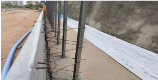
Figure 10. Laying geotextile on a crushed stone base layer 图 10. 碎石垫层铺设土工布
