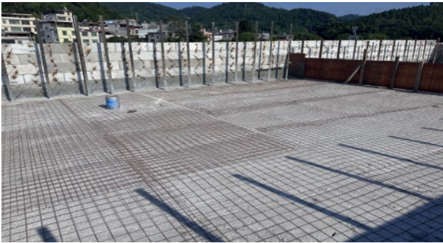
Figure 15. Foam lightweight concrete reinforcement mesh installation 图 15. 泡沫轻质混凝土钢筋网设置
