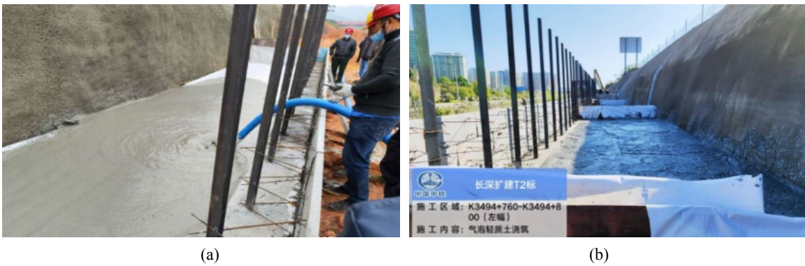
Figure 14. Foam lightweight concrete on-site pouring diagram 图 14. 泡沫轻质混凝土现场浇筑图
