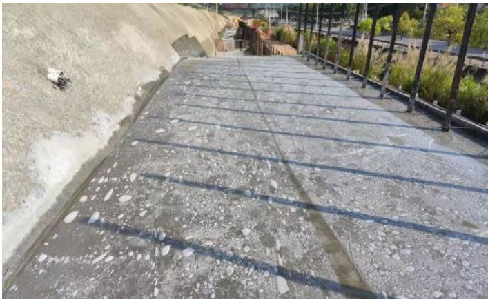
Figure 1. Curing of finished foam lightweight concrete products 图 1. 泡沫轻质混凝土成品养护
