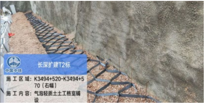
Figure 9. Foam lightweight concrete geocell installation 图 9. 泡沫轻质混凝土土工格室铺设
