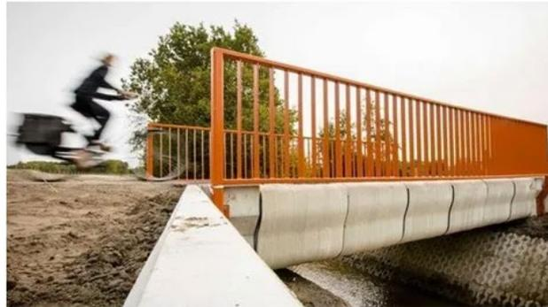
Figure 6. 3D printed bicycle bridge in Eindhoven, Netherlands
