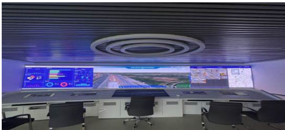
Figure 18. Video surveillance and slope monitoring data are uploaded to the owner's integrated platform from time to time
