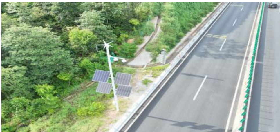
Figure 17. Slope surveillance camera
