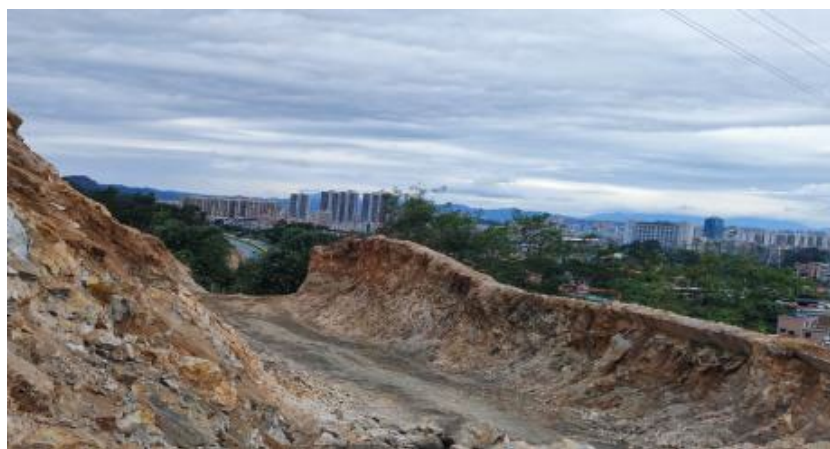
Figure 8. Construction of a central walkway and a reserved slag retaining wall
