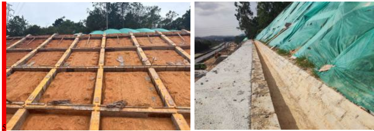
Figure 10. Anchor cable frame beam protection and platform drainage ditch 图 10. 施作锚索框格梁防护及平台排水沟
