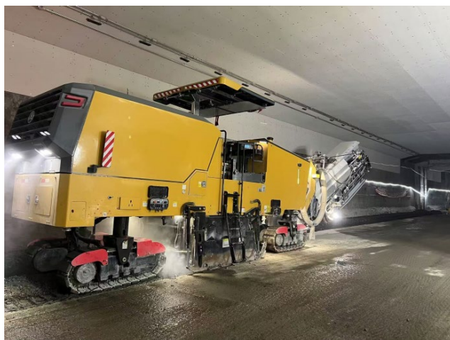
Figure 3. Concrete pavement milling equipment
