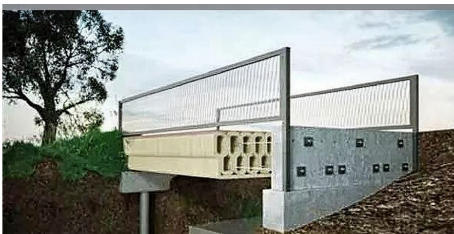
Figure 4. The world's first 3D printed prestressed bicycle bridge 图 4. 全球首座 3D 打印预应力自行车桥
