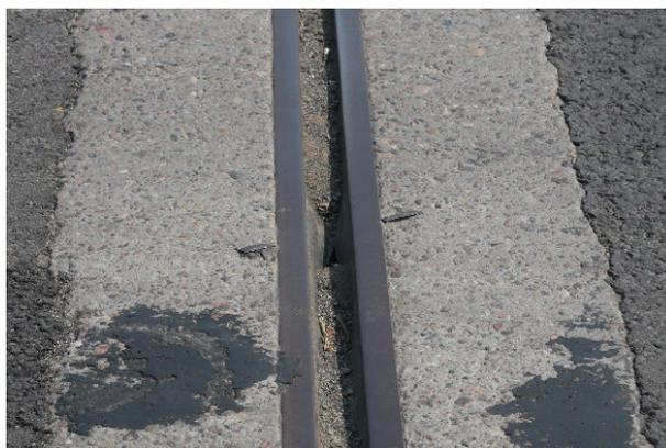
Figure 2. The waterstop of the expansion joint is broken
