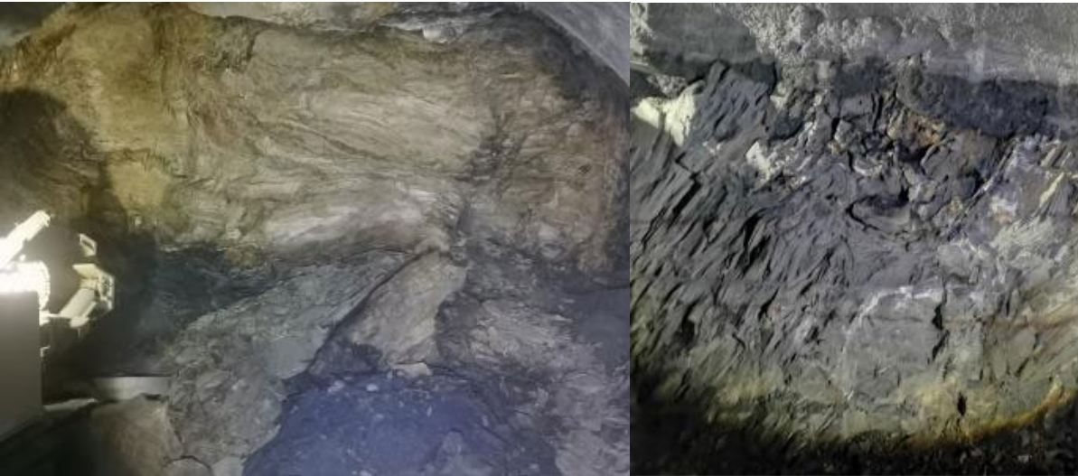
Figure 1. Photos of the tunnel face and side walls of a highway tunnel with Grade V surrounding rock 图 1. 某公路隧道 V 级围岩掌子面和边墙照片
