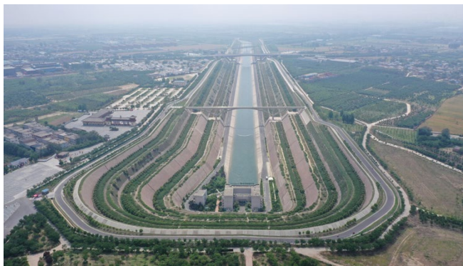
Figure 1. Aerial photo of the south-to-north water diversion project in Zhengzhou, Henan Province, China 图 1. 河南郑州航拍南水北调穿黄工程
