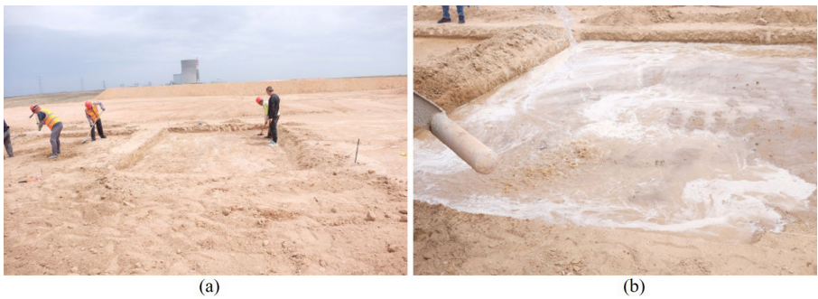
Figure 2. Ground preprocessing: (a) ground leveling; (b) water injection to moisten 图 2. 地面预处理: (a) 地面整平; (b) 注水润湿
