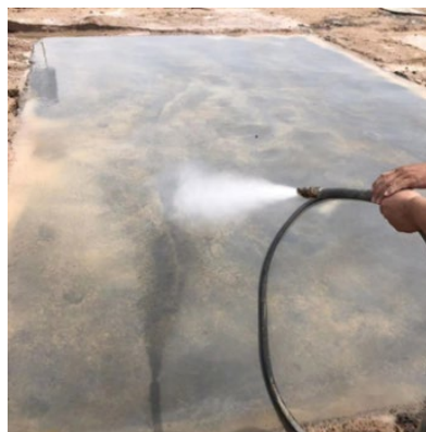
Figure 5. Regular moisturizing maintenance 图 5. 定期湿润养护
