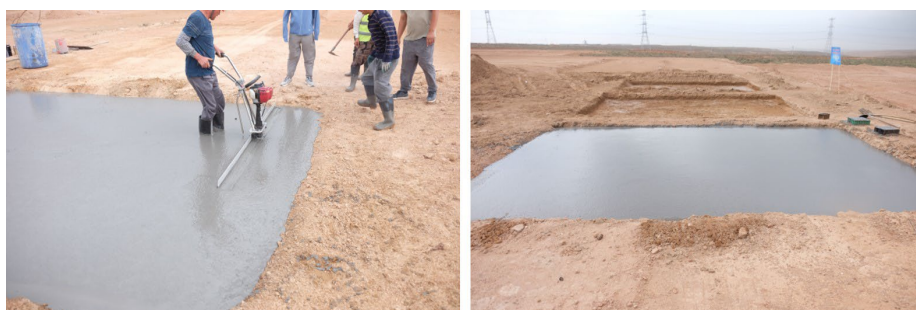
Figure 4. Vibration smoothing of test section 图 4. 试验段振动抹平
