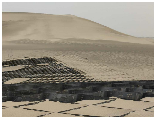
Figure 4. Sand fixation with Geocells
