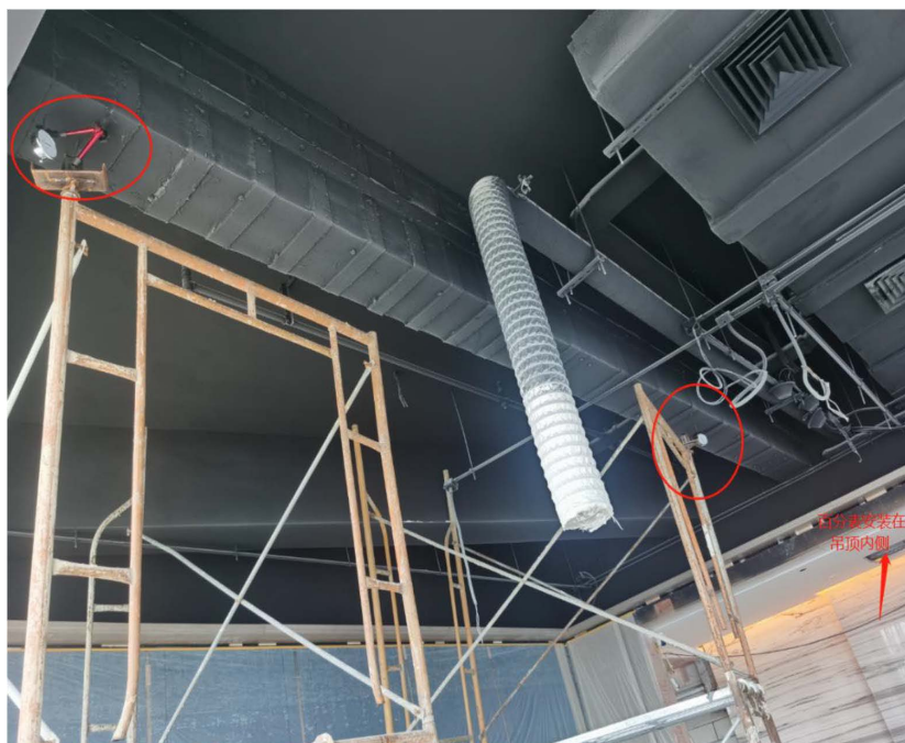
Figure 4. On-site layout diagram of measuring points
