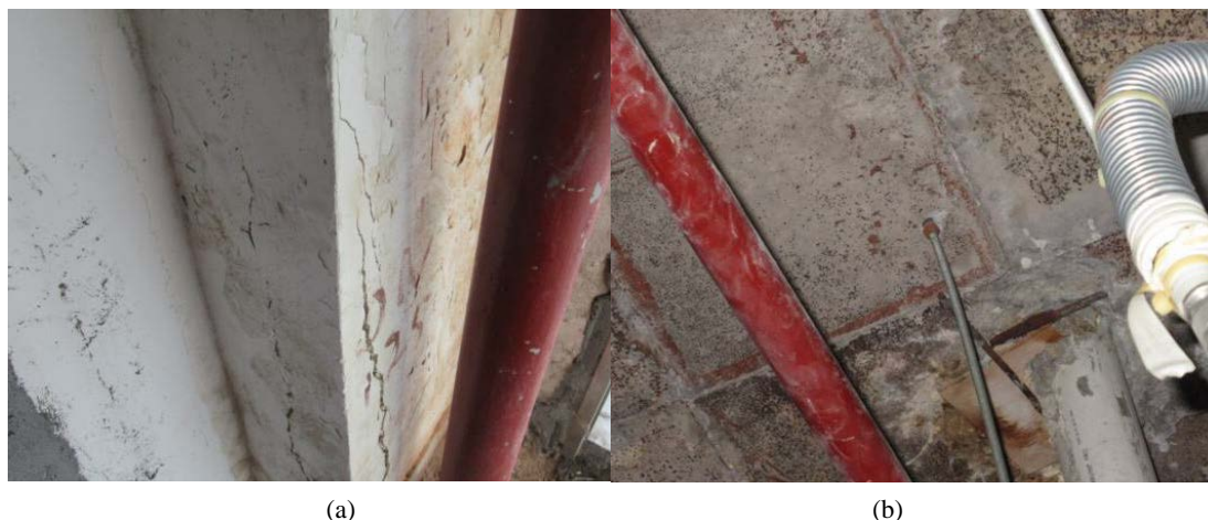
Figure 2. On-site survey drawing, (a) Cracking, water seepage and yellowing; (b) Spalling of protective layer and corrosion of steel bars in concrete slabs
