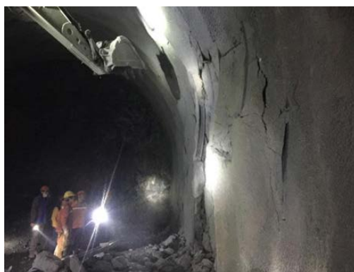
Figure 1. Rockburst hazard in a tunnel 图 1. 隧道岩爆灾害
