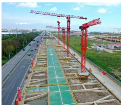
Figure 1. Prefabricated steel trestle 图 1. 装配式钢栈桥
