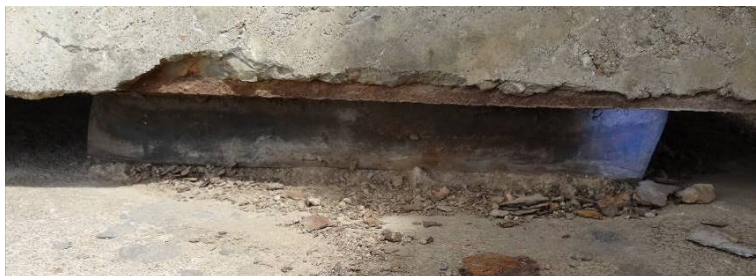
Figure 4. Shear overrun of plate rubber bearing 图 4. 板式橡胶支座剪切超限
