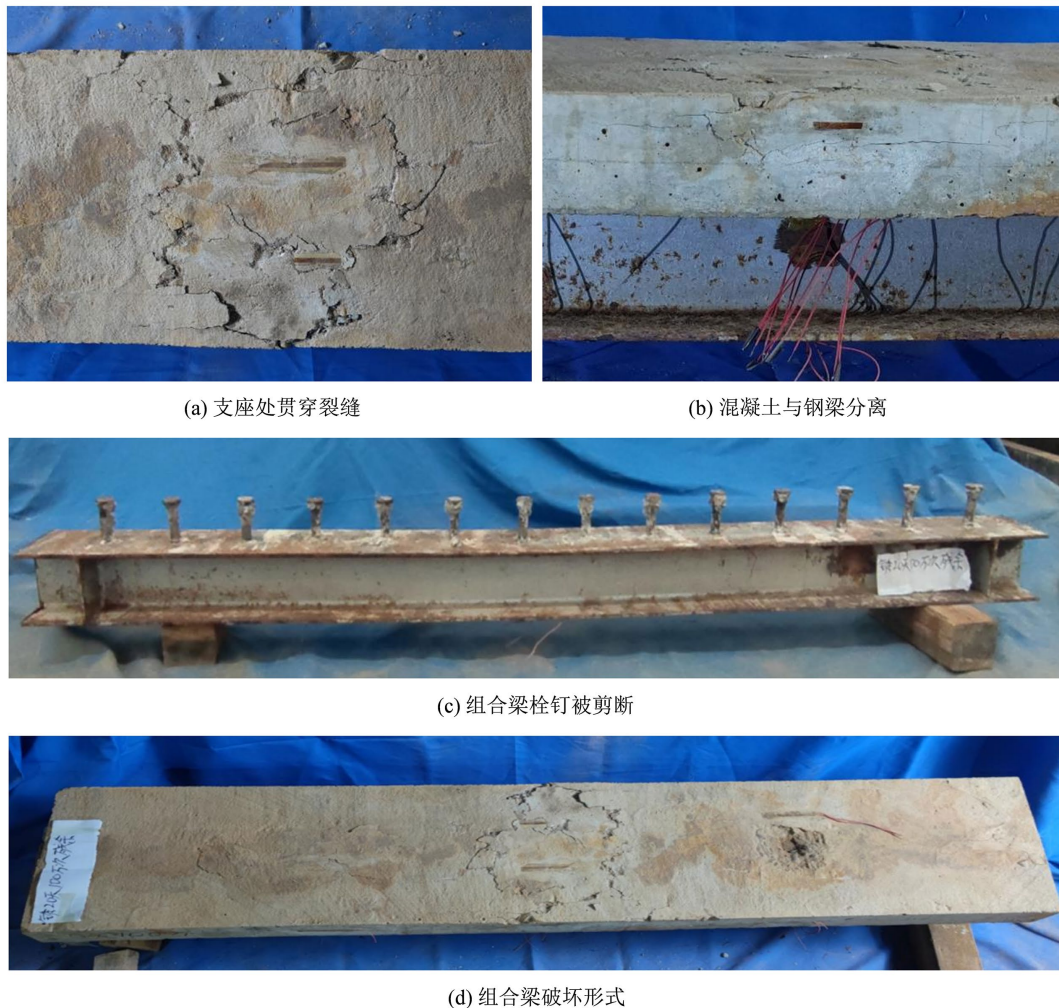
Figure 7. Failure modes of corroded specimens
