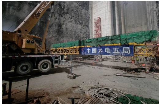
Figure 3. Site photo of slipform assembly 图3. 滑模组装现场图
