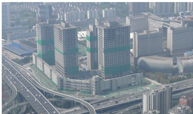
Figure 1. High-rise buildings to be demolished and surrounding environment 图 1. 待拆高层建筑物及周边环境
