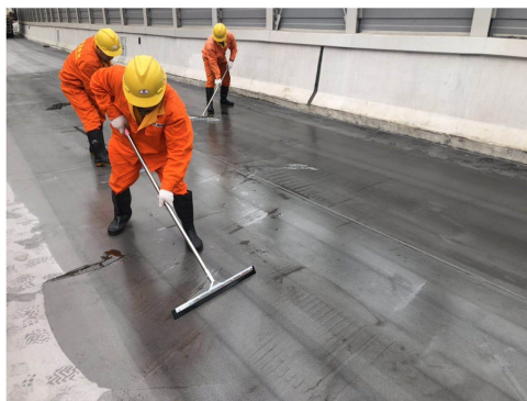
Figure 1. Application of polyurethane waterproof bonding layer on steel bridge deck 图 1. 钢桥面涂刷聚氨酯防水粘结层应用
