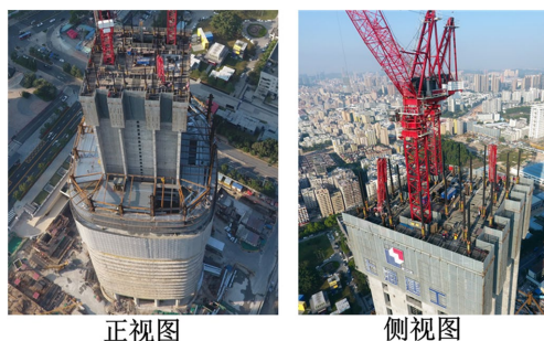
Figure 5. ICCP used in the construction of a 356-meter core wall structure
