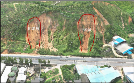
Figure 2. H1 and H2 landslides 图 2. H1，H2 滑坡
