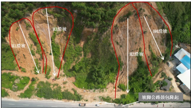
Figure 3. H3 and H4 landslides 图 3. H3, H4 滑坡
