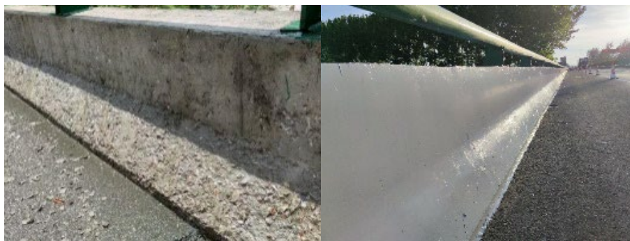
Figure 1. Comparison of concrete barrier before and after coating construction
