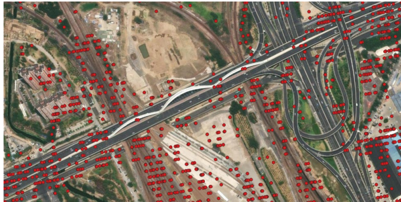
Figure 4. Distribution of PS points near Caihong Bridge 图 4. 彩虹桥附近 PS 点分布情况
