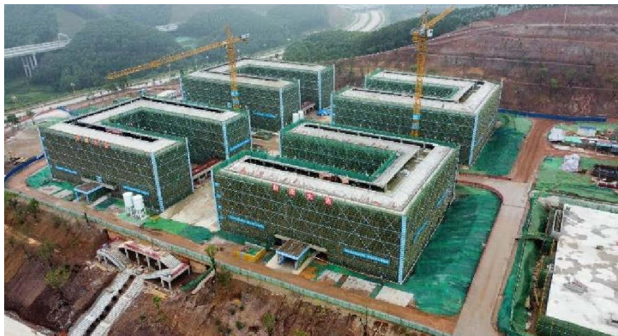
Figure 2. Construction site dust control 图2. 施工现场扬尘管控
