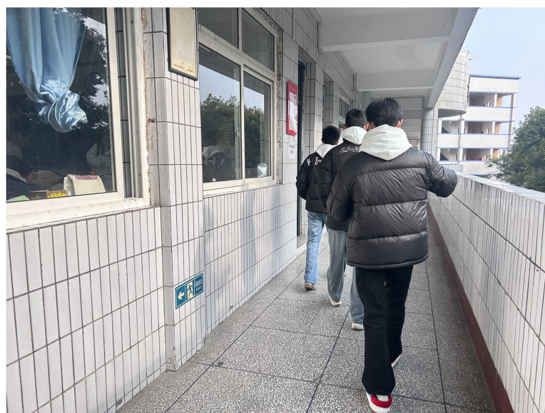
Figure 3. The balustrades are enclosed (Photo taken by the author)
