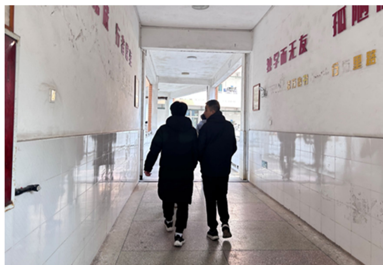
Figure 2. The connecting corridor is poorly lit (Photo taken by the author)
