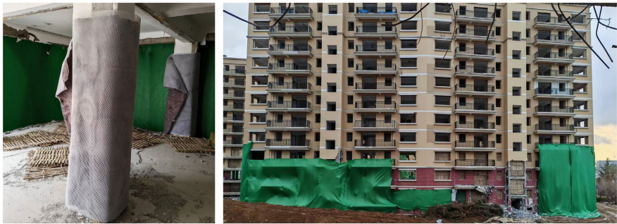
Figure 11. Protection for blasting areas 图 11. 爆破部位防护
