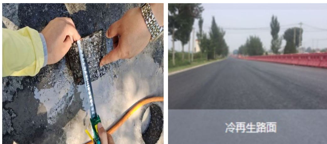
Figure 5. Field application of foamed asphalt cold recycled pavement 图 5. 泡沫沥青冷再生路面实施效果图
