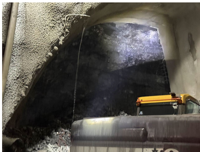
Figure 1. Photos of the construction site of the tunnel
