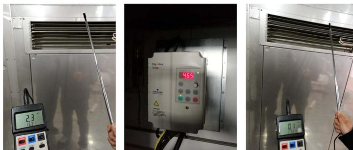
**Figure 3. Result of airflow adjustment**
