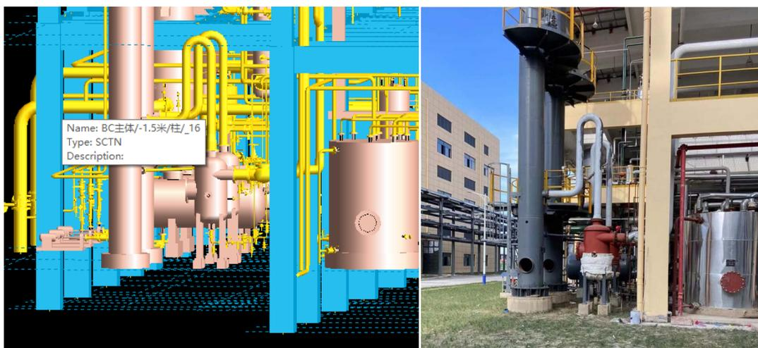
Figure 1. Comparison between PDMS model and on-site installation effect
