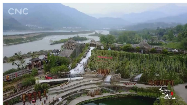
Figure 11. The aerial view of Min River and irrigation zone
