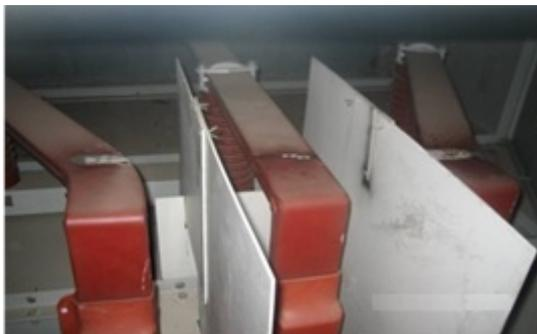
Figure 1. The distribution of bus and insulating barrier in 35 kV switchgear
