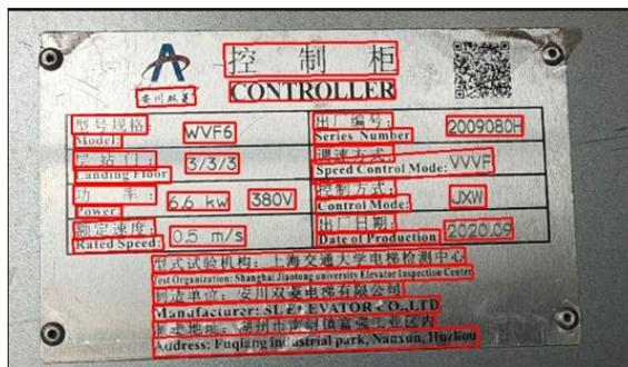
Figure 9. Elevator nameplate character detection results
