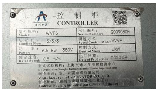
Figure 8. Elevator nameplate number
