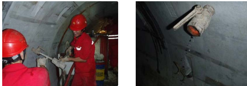
Figure 3. The inspection of grouting effect through grouting hole of the segment
