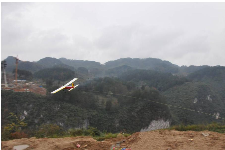
Figure 6. Model drawing pilot rope across the river
