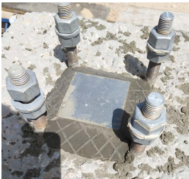
Figure 5. Shim plate installation 图 5. 坐浆板安装
