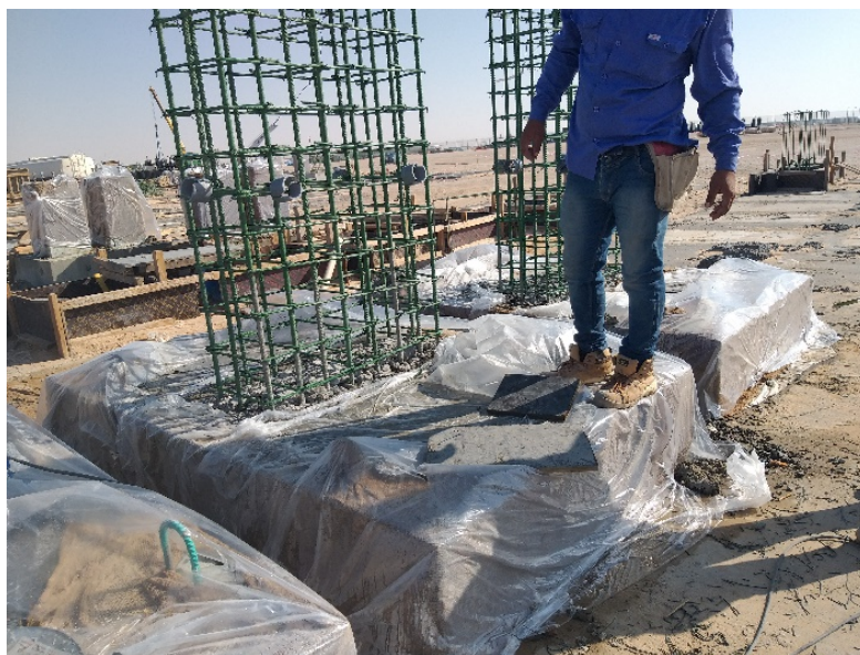
Figure 2. Foundation cast in layers 图 2. 分层浇筑的基础
