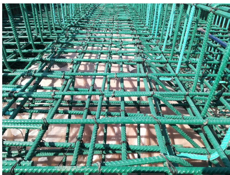
Figure 1. Rebar binding
