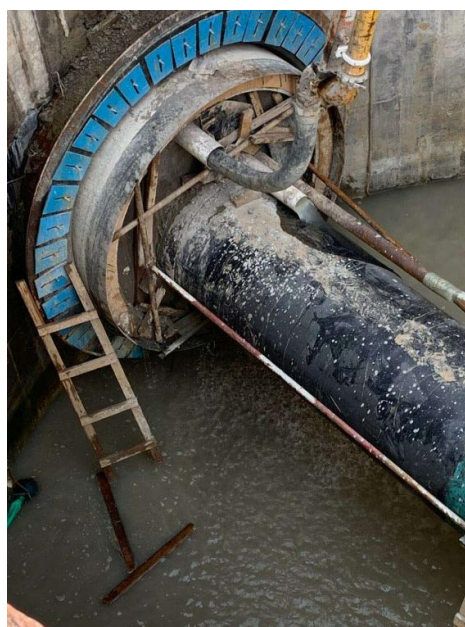
Figure 3. Filling of cement mortar on site casing
