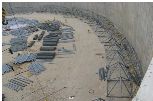
Figure 1. Live assembly of module
