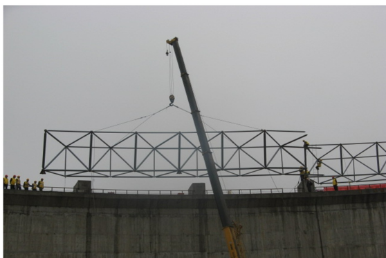
Figure 5. Reticulated shell docking of the second hoisting unit 图 5. 网架第二吊装单元对接
