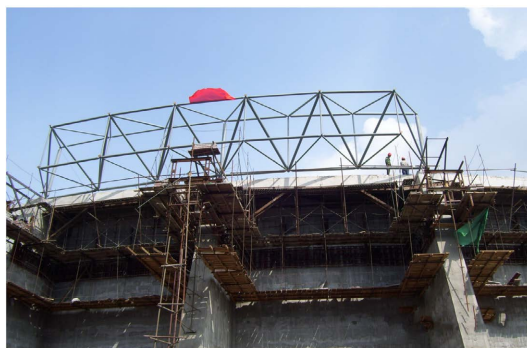
Figure 4. The first hoisting unit of the reticulated shell is hoisted in place
