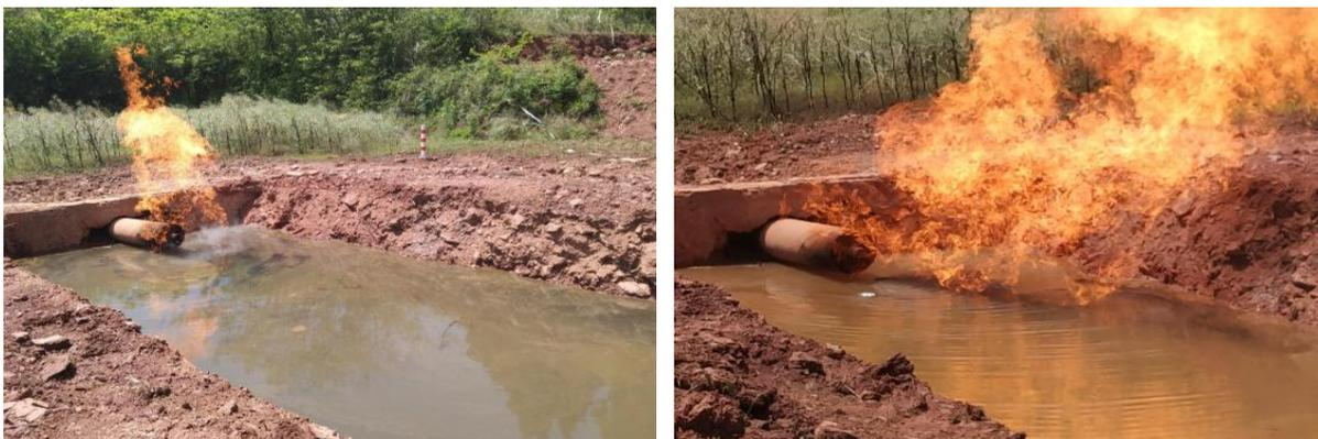
Figure 2. Blowout at the second stage of well M-AH29 plugging removal
