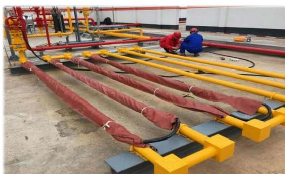
Figure 3. Electric heating device
