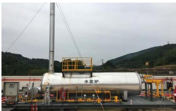
Figure 2. Water jacket heating furnace
