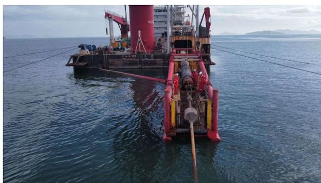
Figure 7. Directional drilling rig towing landing and bottom hole assembly (BHA)
