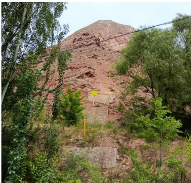
**Figure 4.** On-site effect diagram of slope bottom retaining wall + steep slope pouring
