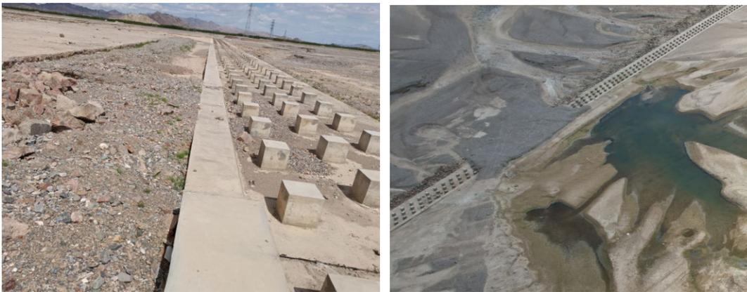
**Figure 8.** On-site effect diagram of concrete anti-scour wall + concrete apron downstream of the anti-scour wall + stilling pier
