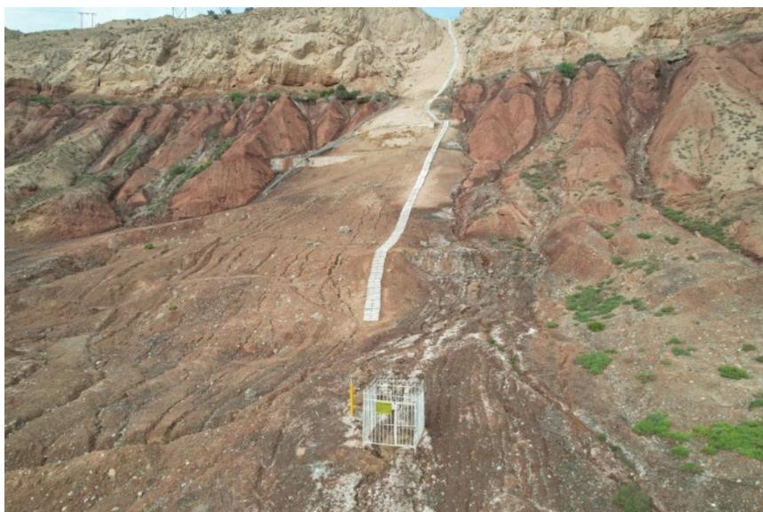
**Figure 3.** On-site effect diagram of slope bottom retaining wall + cut-off wall + drainage ditch
