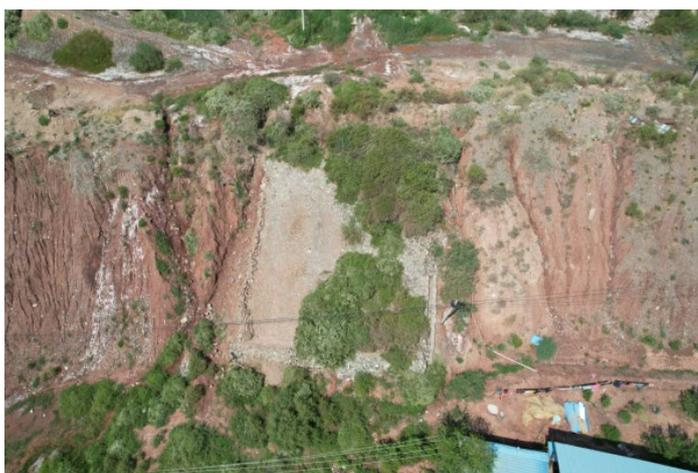
**Figure 1.** On-site effect diagram of dry stone retaining wall at slope foot + mortar stone slope protection + longitudinal drainage ditch on slope surface in loess steep slope area
