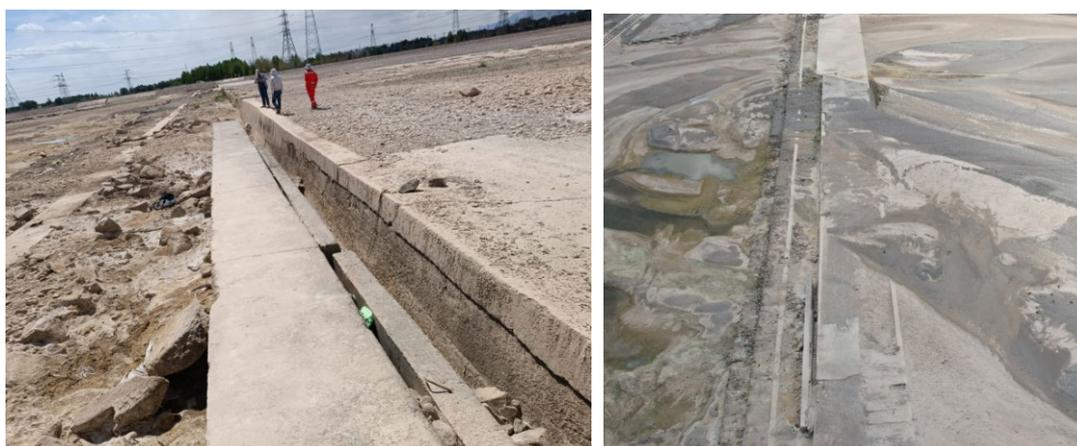
**Figure 7.** On-site effect diagram of anti-scour wall + concrete overflow surface + three-stage gabion apron
