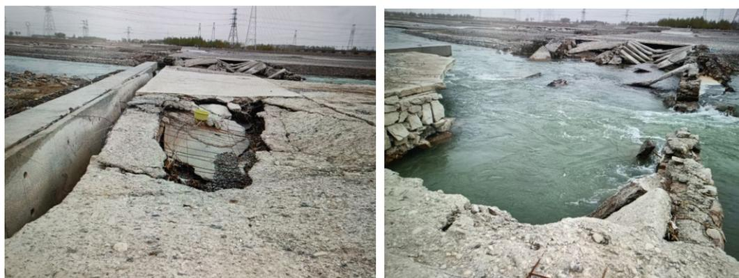
**Figure 6.** On-site effect diagram of anti-scour wall + reinforced concrete overflow surface between anti-scour walls + gabion apron downstream of anti-scour wall
