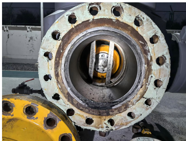
Figure 2. Detector receiving 图 2. 检测器收球后情况
