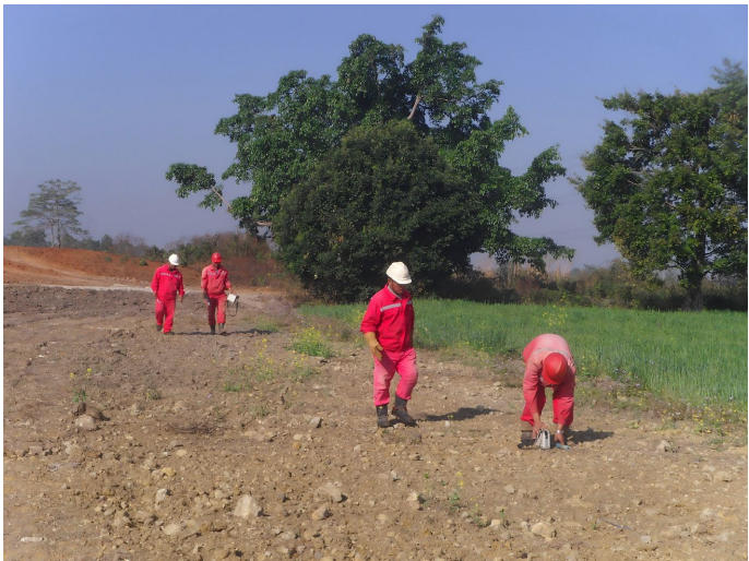
Figure 9. Picture of tracking the diameter gauging pig with a pipeline tracker 图 9. 利用跟踪仪跟踪测径清管器照片
