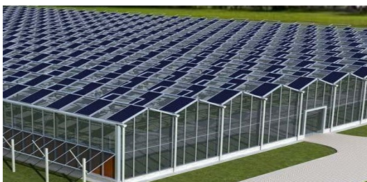
Figure 3. Photovoltaic shed 图 3. 光伏大棚
