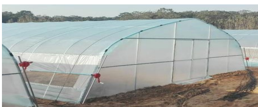
Figure 1. Arch shed 图 1. 单体拱棚
