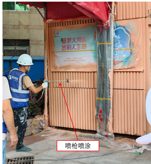
Figure 1. On-site construction of passive radiative cooling coating 图 1. 被动辐射制冷涂层现场施工
