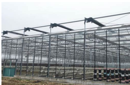
Figure 7. Physical picture of tempered glass frame structure 图 7. 钢化玻璃钢架结构实物图
