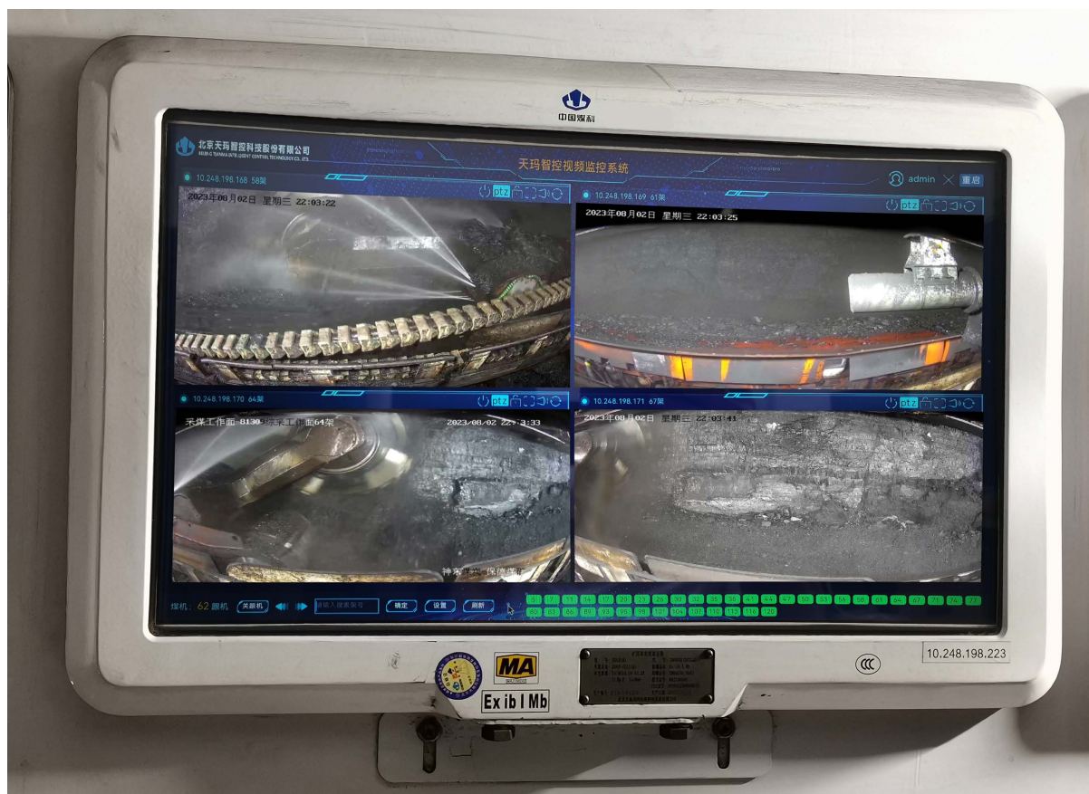
Figure 7. Integrated machine display images in coal mine
