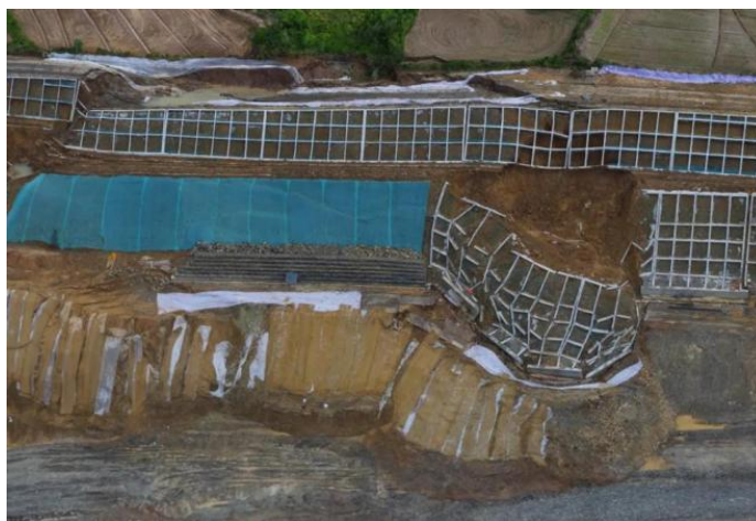
Figure 2. Image of landslide mass in J6-J7 section of the south slope of the mining area
