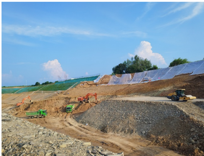
Figure 5. Replacement construction 图 5. 换填施工
