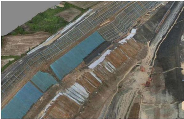
Figure 10. Image of mine boundary slope 图 10. 矿界边坡影像图
