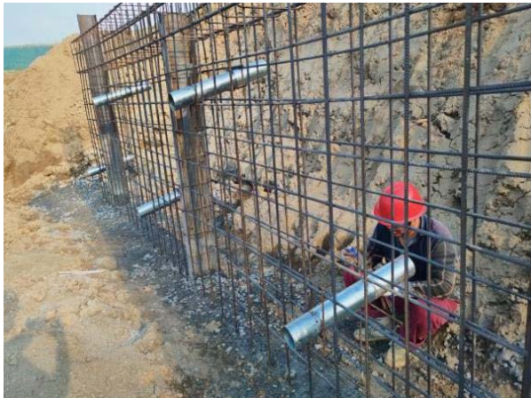
Figure 11. Reinforcement project using micro-anti-slide pile and slab wall 图 11. 微型抗滑桩板墙加固工程
