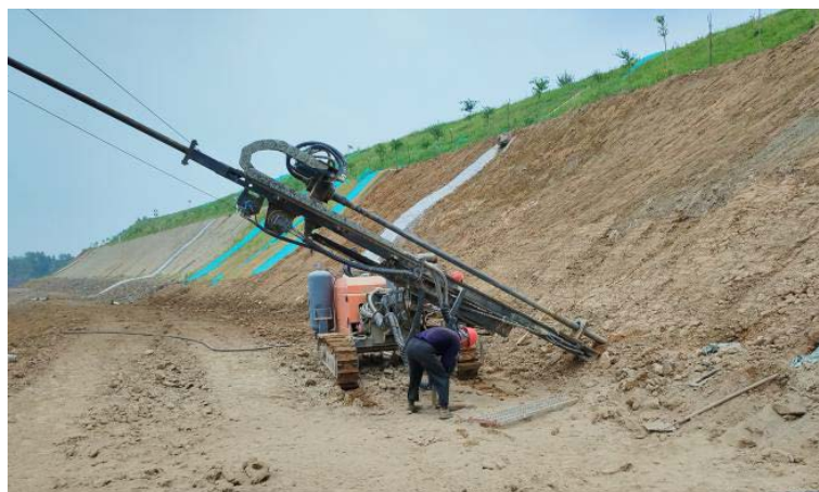
Figure 12. Slope shoulder reinforcement project 图 12. 坡肩加固工程
